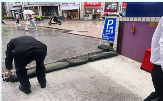
On-site flood management trainings in China include placing sandbags and water blocking gates at building entrances
