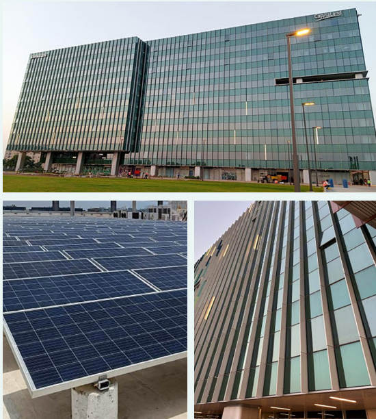
Clockwise from top: International Tech Park Chennai - Radial Road (ITPC-RR) Aluminium fins on external façade of ITPC-RR to reduce solar heat gain and improve thermal comfort Solar panels on rooftop of ITPC-RR
