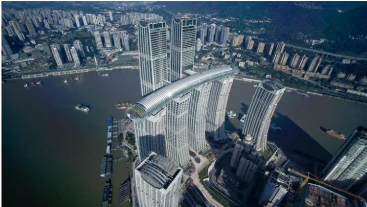
An exterior view of Raffles City Chongqing. The Crystal sky bridge is nestled atop four 250-metre-tall skyscrapers and linked to two adjacent skyscrapers by cantilever bridges.
