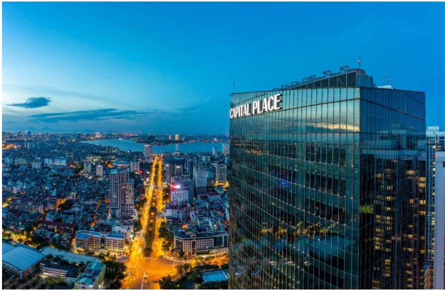
CapitaLand Development divests Capital Place in Hanoi for S$751 million (US$550 million) as part of its capital recycling strategy
