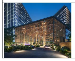
Mass engineered timber (MET) harvested from sustainably managed forests is used to construct the canopies and columns at Geneo's event plaza. When completed, Geneo's 3,000 sq m all-weather event plaza measuring 27 metres in height will be Singapore's tallest MET canopy structure.
