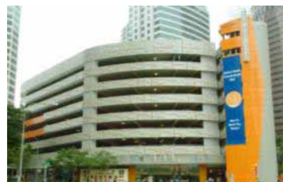
Market Street Car Park, Singapore
