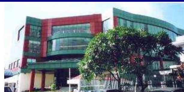
Quill Building 10 – HSBC (Section 13)
