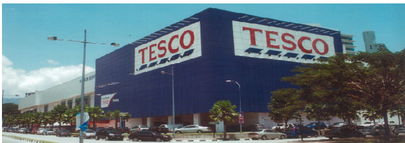
TESCO Building, Penang
