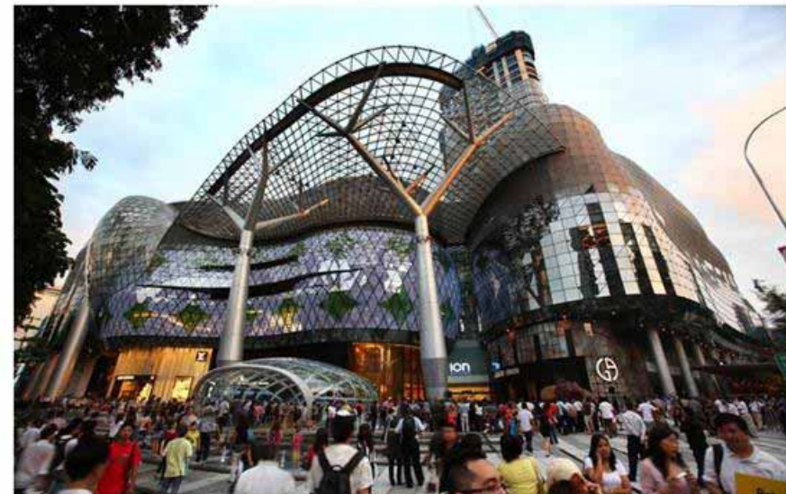
ION Exterior with LED lights
