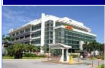
Quill Building 4 - DHL 2
