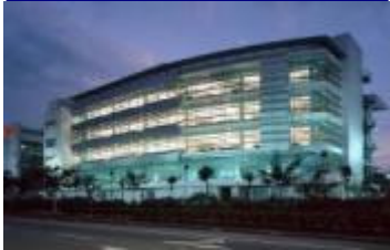
Quill Building 1 - DHL 1
