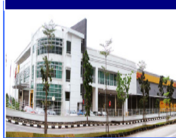
Quill Building 8-DHL (XPJ)
