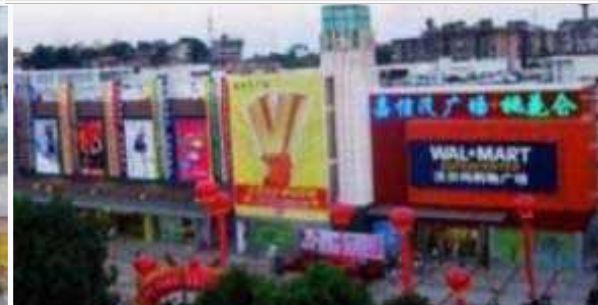
Taohualun Mall, Yiyang Opened on 9 Apr 2009
