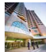
Somerset Olympic Tower Property Tianjin
