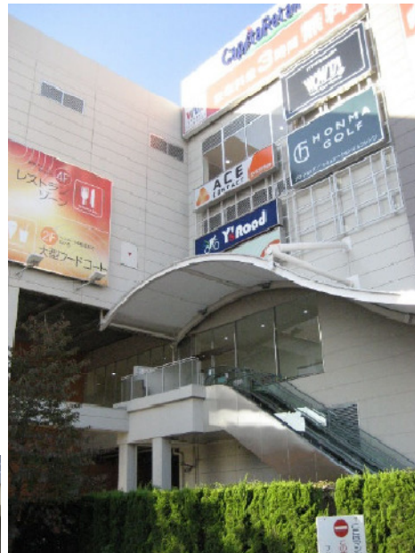
Escalator to 2 nd Flr
