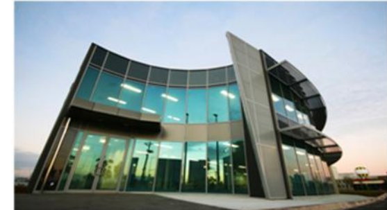
Greens Road, Dandenong, Victoria
