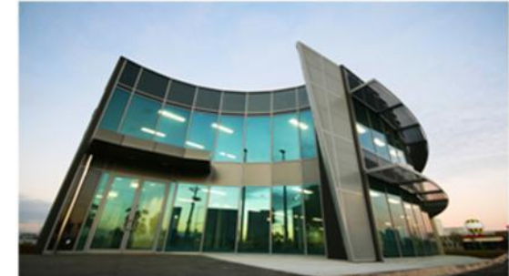
Greens Road, Dandenong, Victoria
