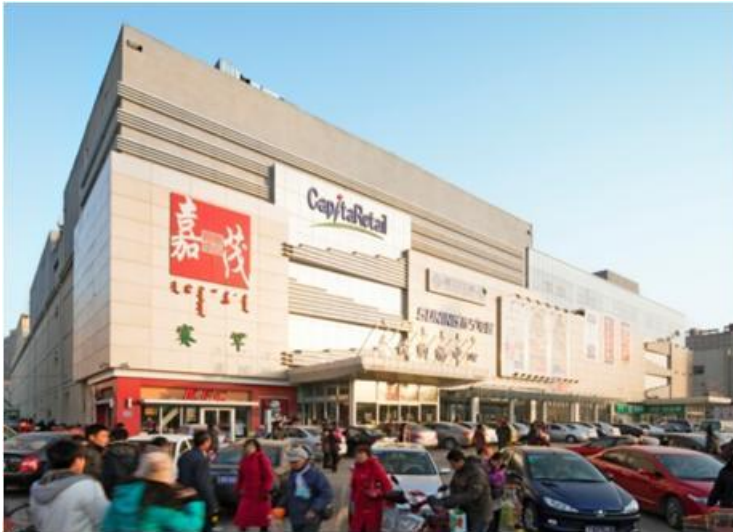
New façade of Saihan Mall
