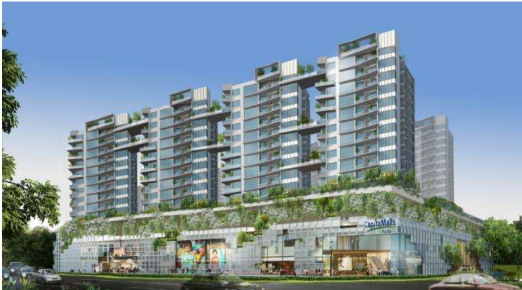
~ 500-unit residential development in Bedok Town Centre
