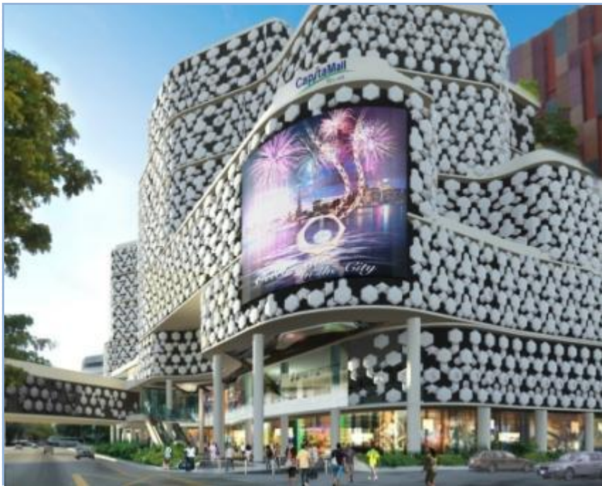
New Facade with LED Screen
