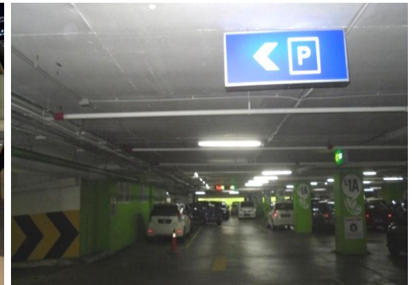
Installation of energy efficient lighting
