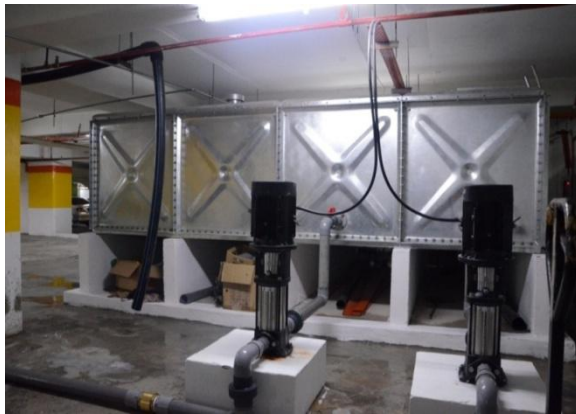
Installation of water recycling tank
