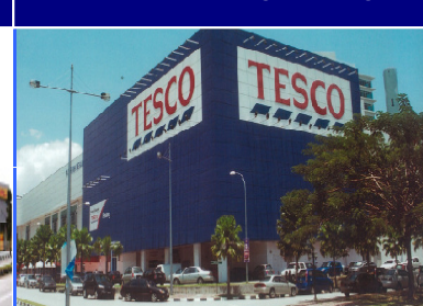
TESCO Building Penang
