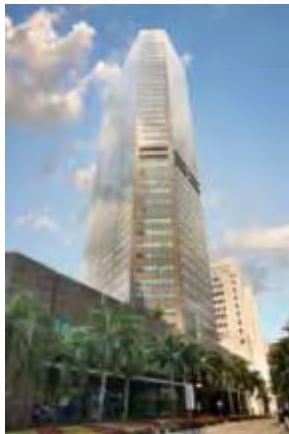
Six Battery Road
