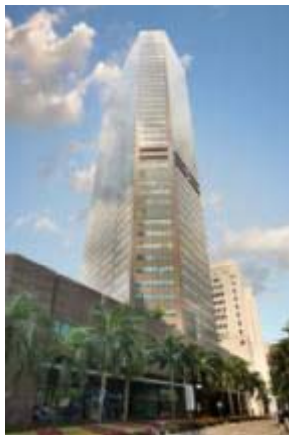
Six Battery Road
