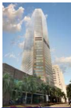
Six Battery Road
