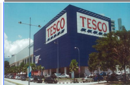
TESCO Building Penang
