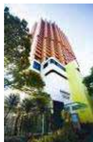
Somerset Liang Court Property
