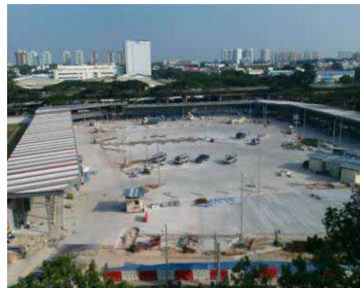
Temporary bus interchange under construction
