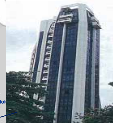
Existing Marine Point building to be redeveloped
