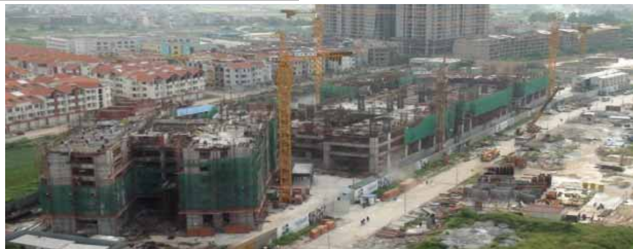
Construction of superstructure in progress
