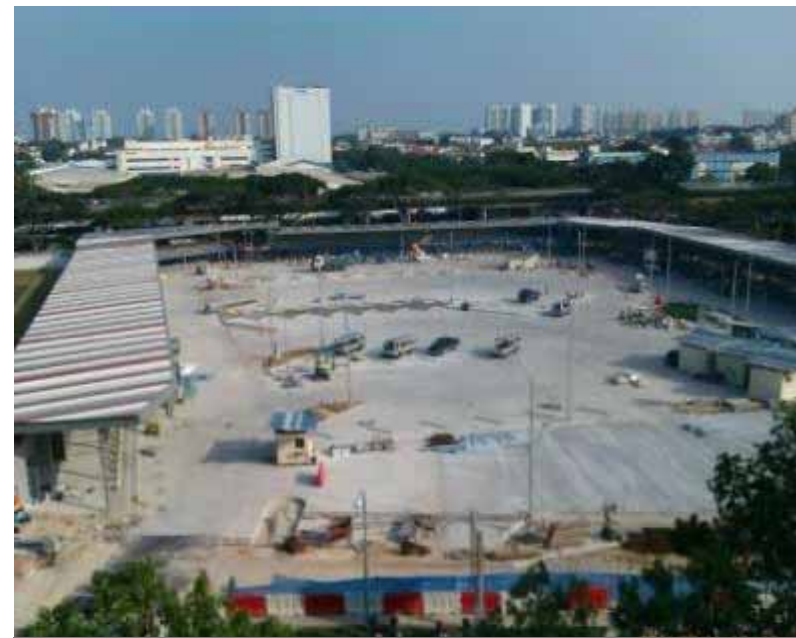
Temporary bus interchange under construction
