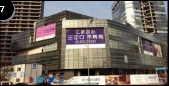
Raffles City Ningbo, Ningbo
