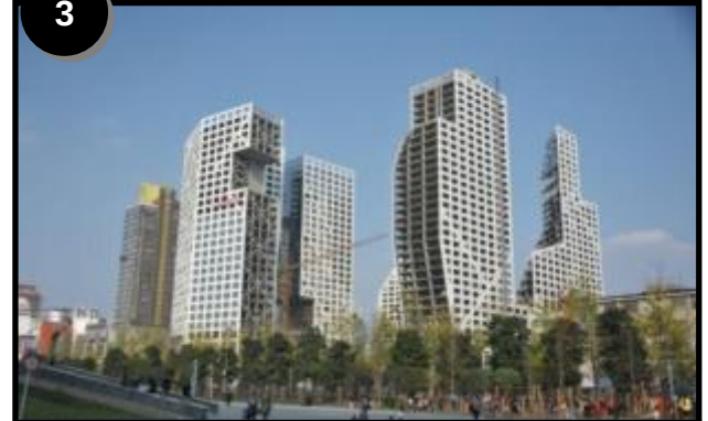
Raffles City Chengdu, Chengdu
