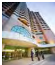
Somerset Olympic Tower Property Tianjin
