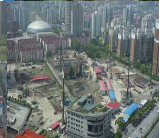
Raffles City Changning, Opening 2015
