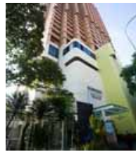
Somerset Liang Court Property
