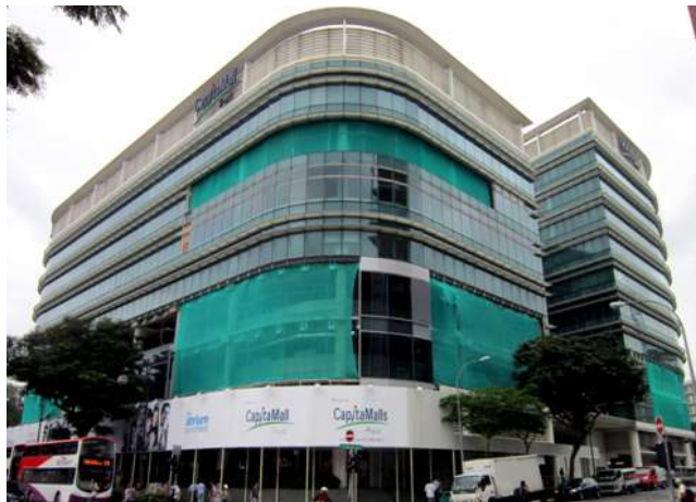
Facade works along Orchard Road
