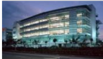
Quill Building 1 - DHL 1
