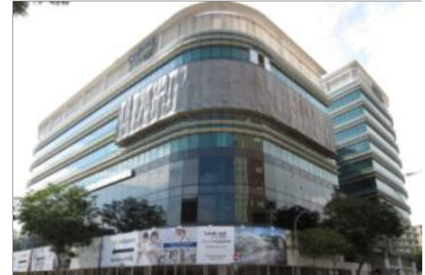
Facade works along Orchard Road
