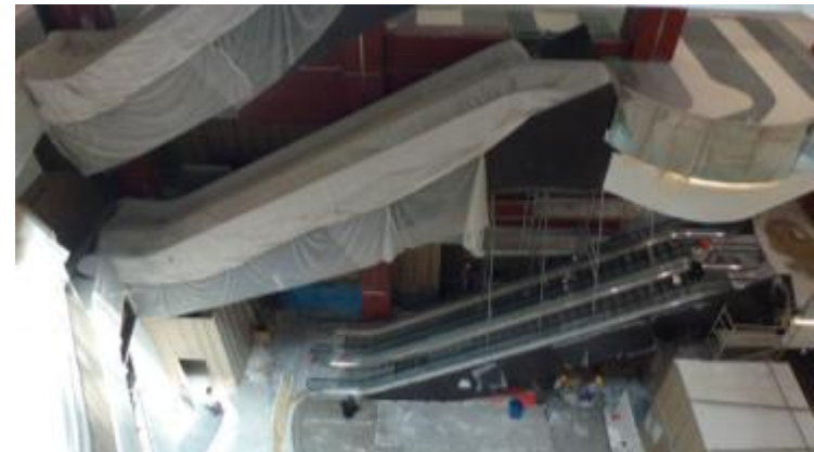
Relocation of escalators for levels 1, 2 and 3
