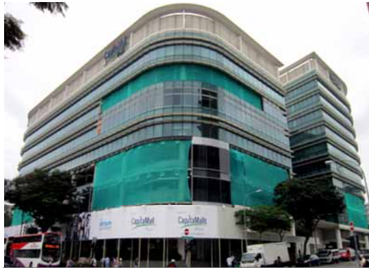
Facade works along Orchard Road
