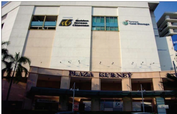
Before repainting of building facade
