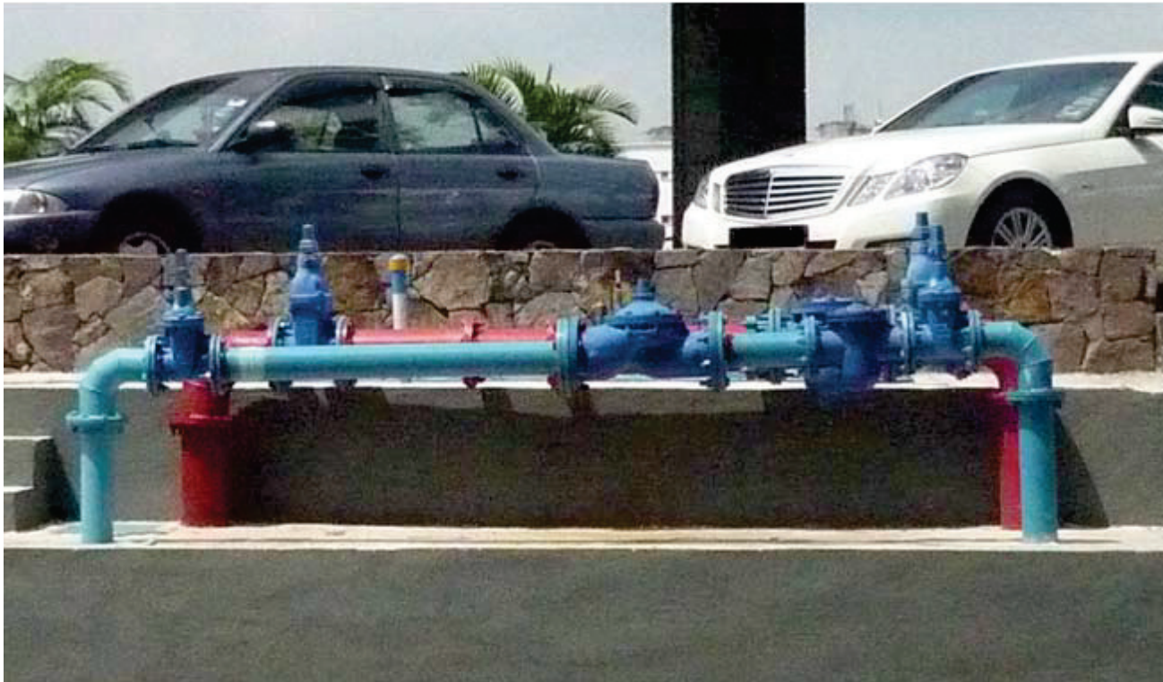
Installation of direct water supply from Syabas
