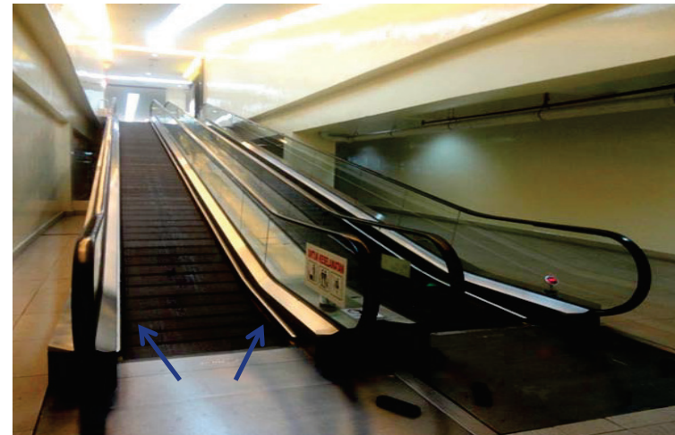
Installation of skirt brushes for travellers
