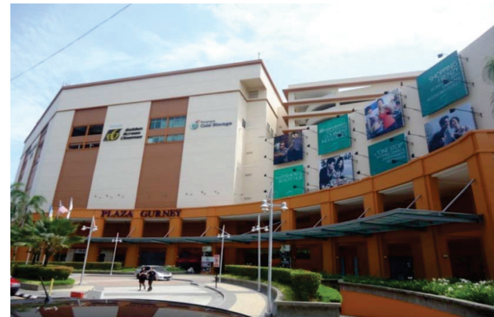
After repainting of building facade
