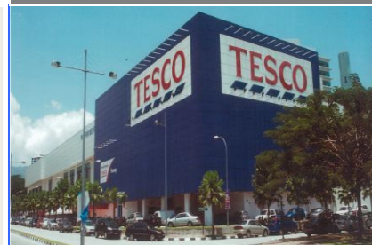
TESCO Building Penang
