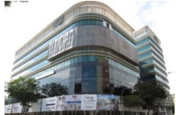
Facade works along Orchard Road
