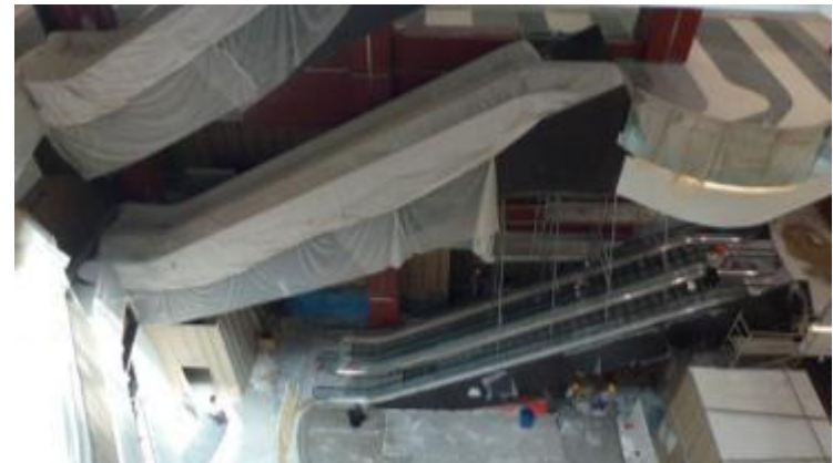
Relocation of escalators for levels 1, 2 and 3
