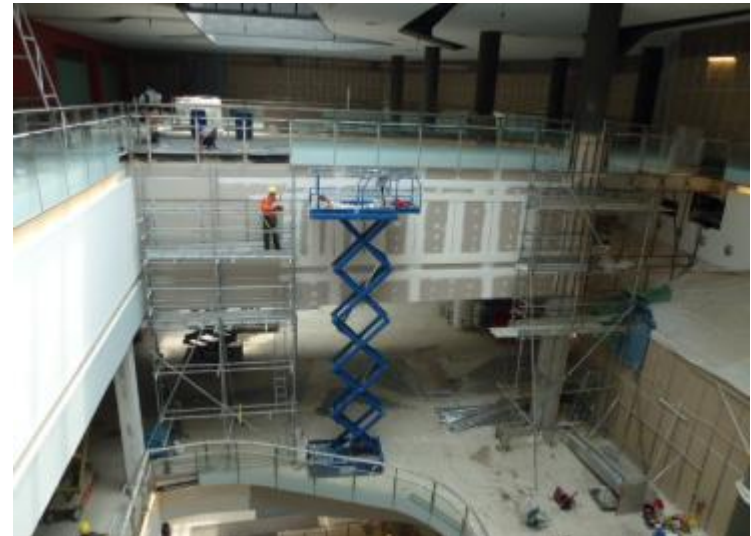
New floor space created on level 5
