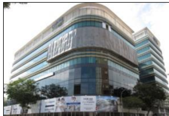
Facade works along Orchard Road
