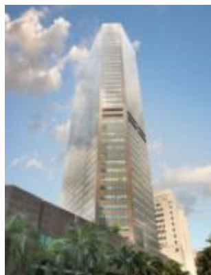
Six Battery Road
