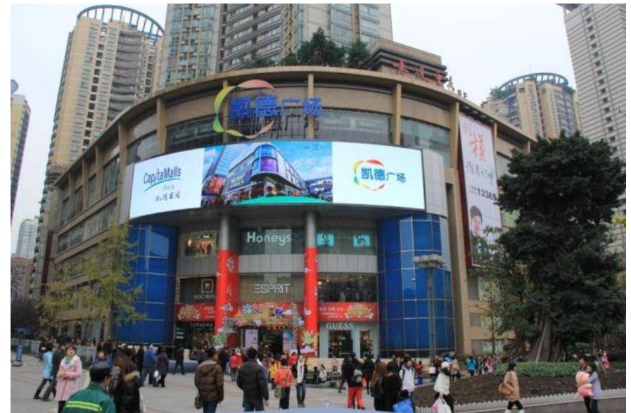
CapitaMall Shapingba, Chongqing
