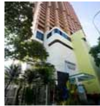
Somerset Liang Court Property
