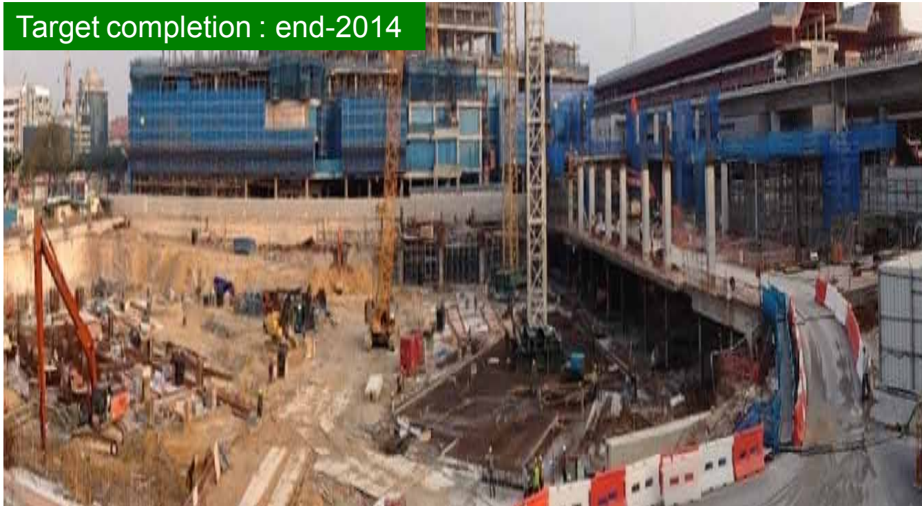
Westgate Tower - Piling Work in Progress
