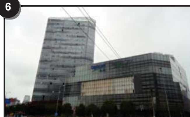
Raffles City Ningbo, Ningbo
