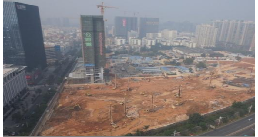
Excavation and shoring system in progress
