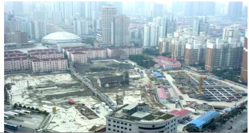
Excavation & shoring system, 12% project completion (steel binding and concrete casting) in progress
