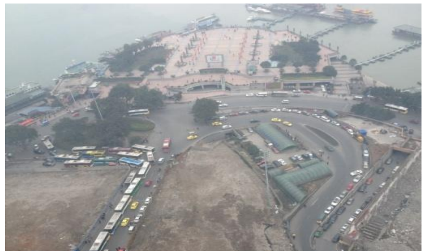
Land resettlement in parallel with design works
