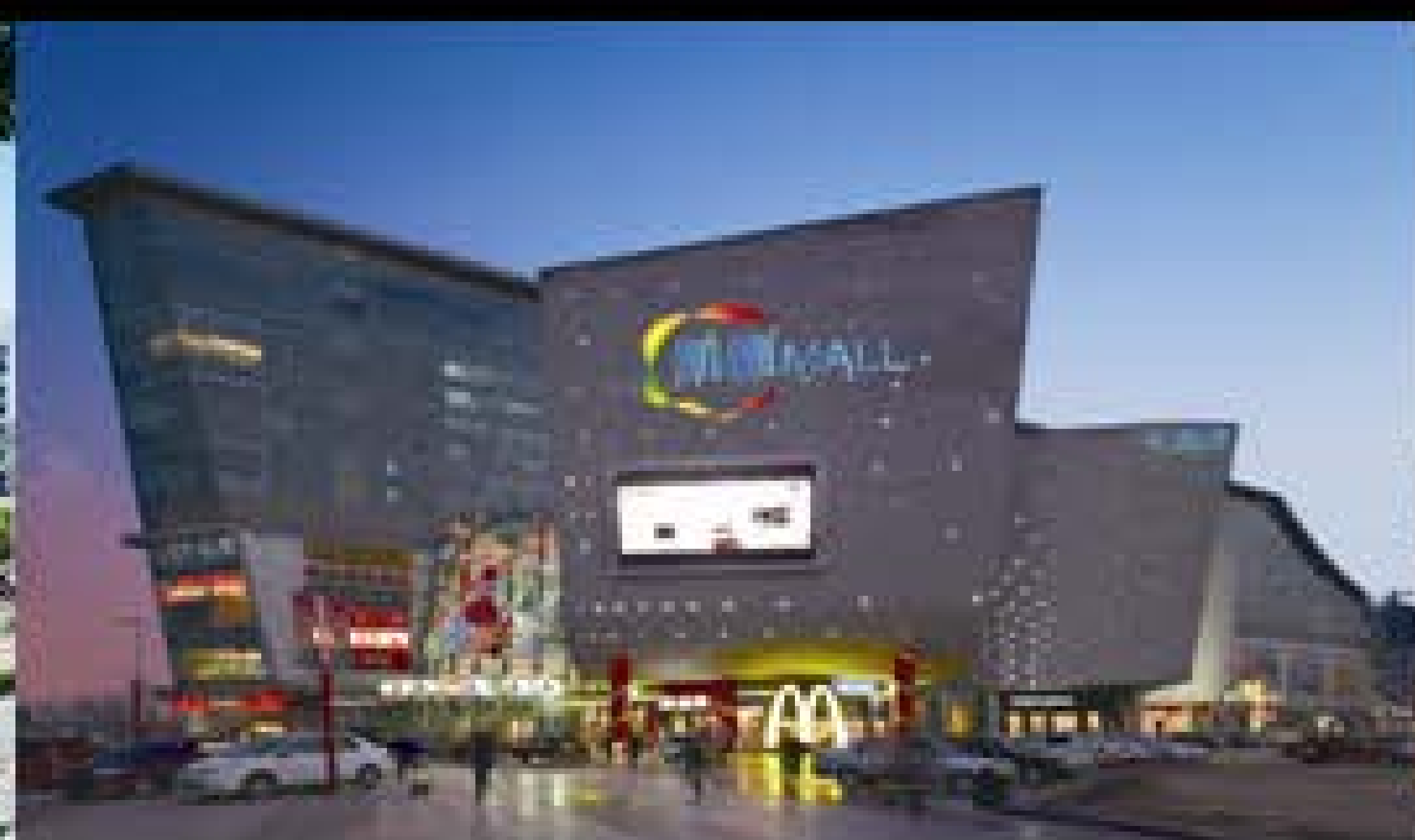
CapitaMall TianjinOne, Tianjin
