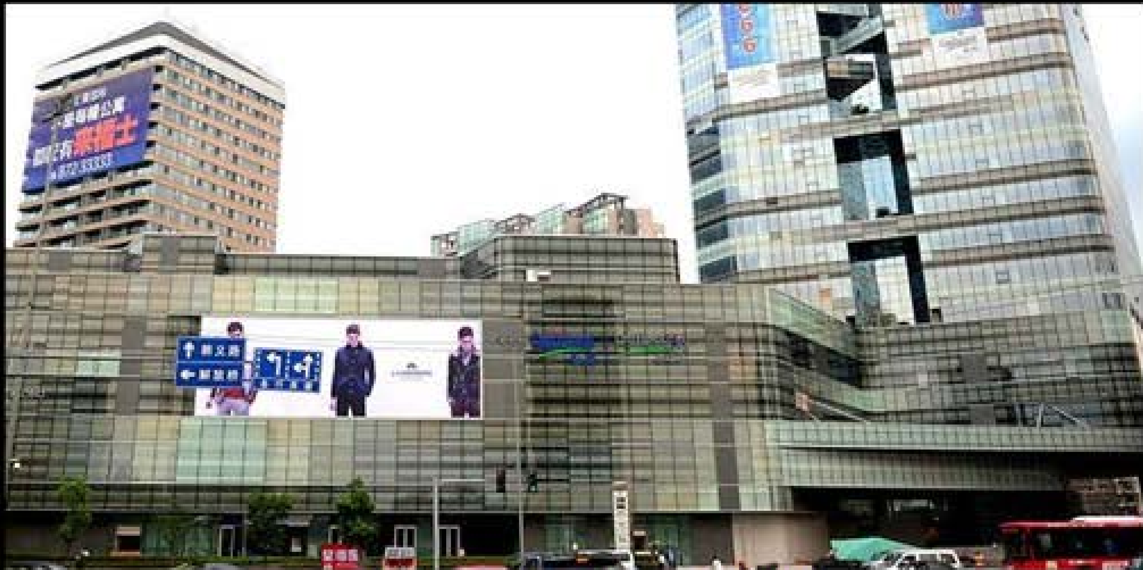
7. Raffles City Ningbo, Ningbo
