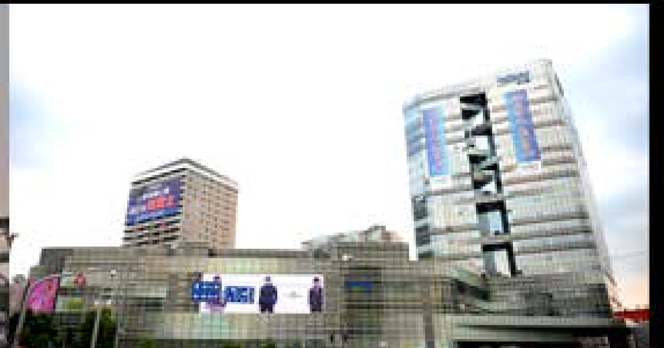
Raffles City Ningbo, Ningbo
