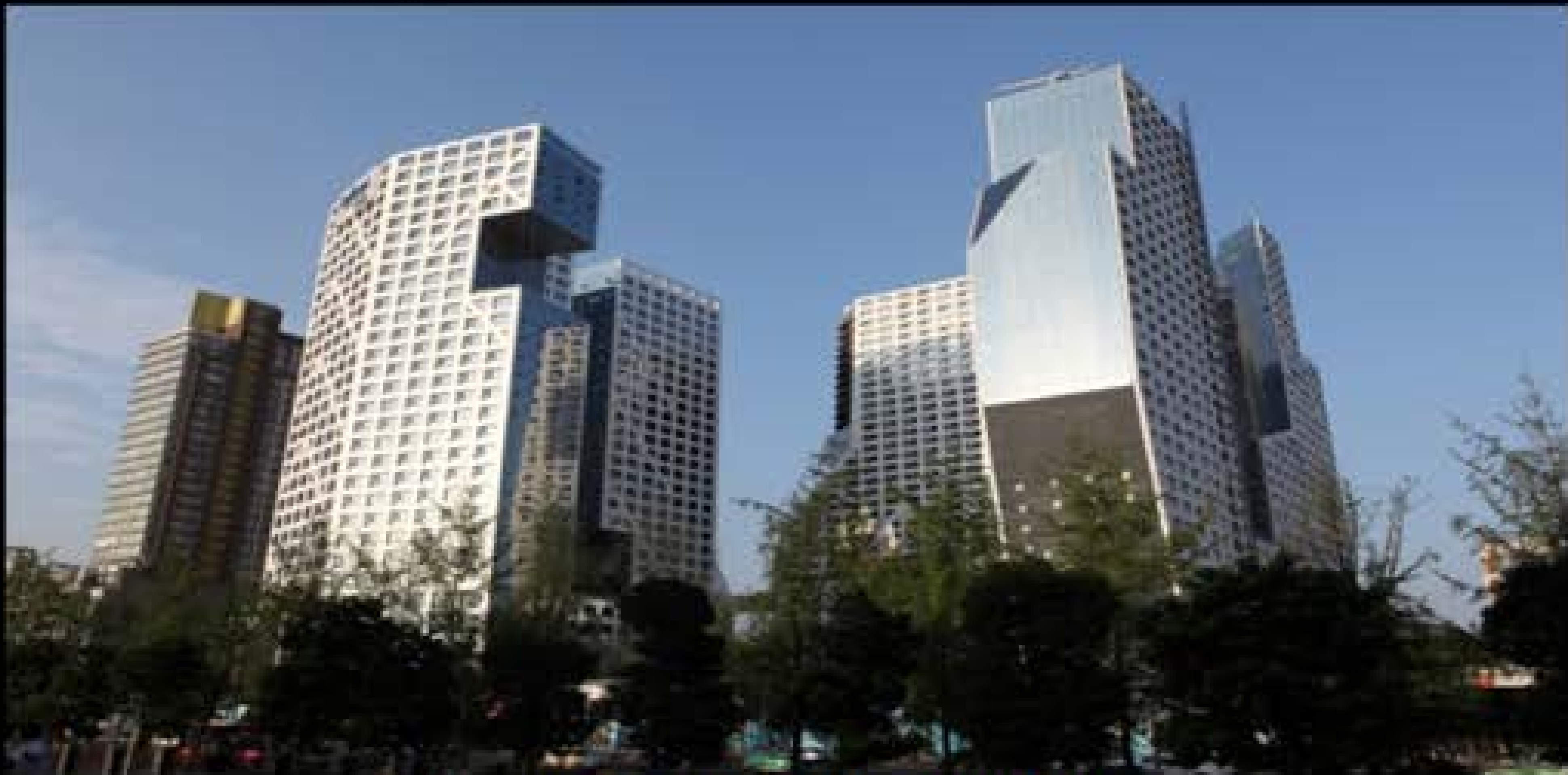
6. Raffles City Chengdu, Chengdu
