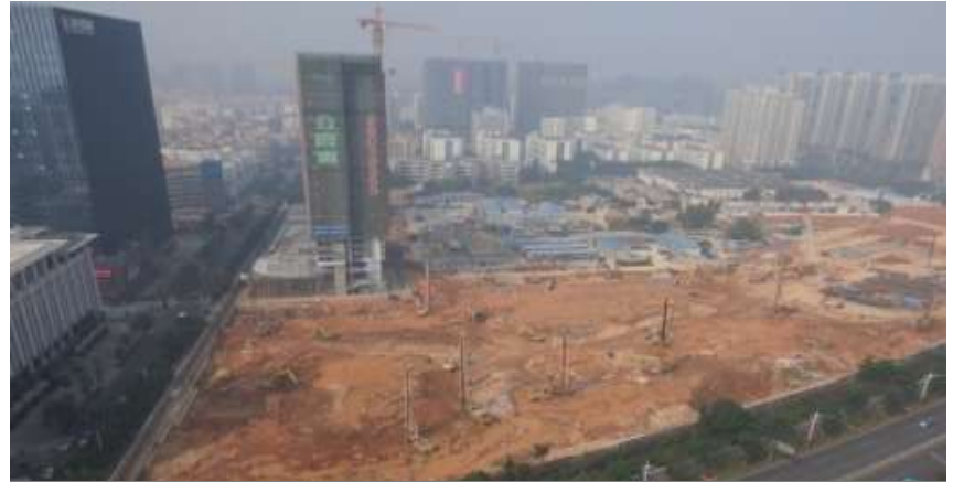
Excavation and shoring system in progress
