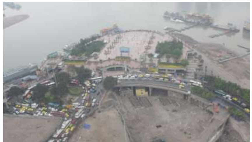
Site clearance in progress
