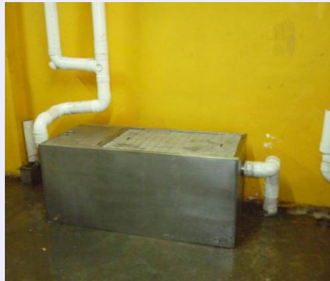
New Grease Trap for Loading Bay 2
