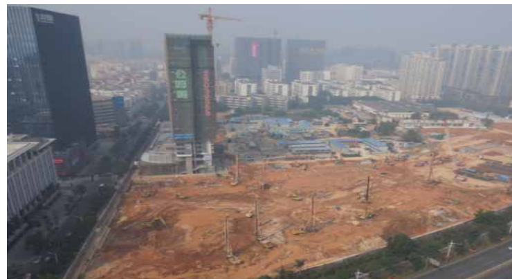
Excavation and shoring system in progress
