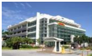
Quill Building 4 - DHL 2
