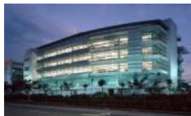
Quill Building 1 - DHL 1
