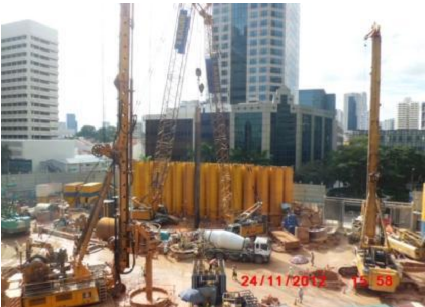
General view of the progress on site
