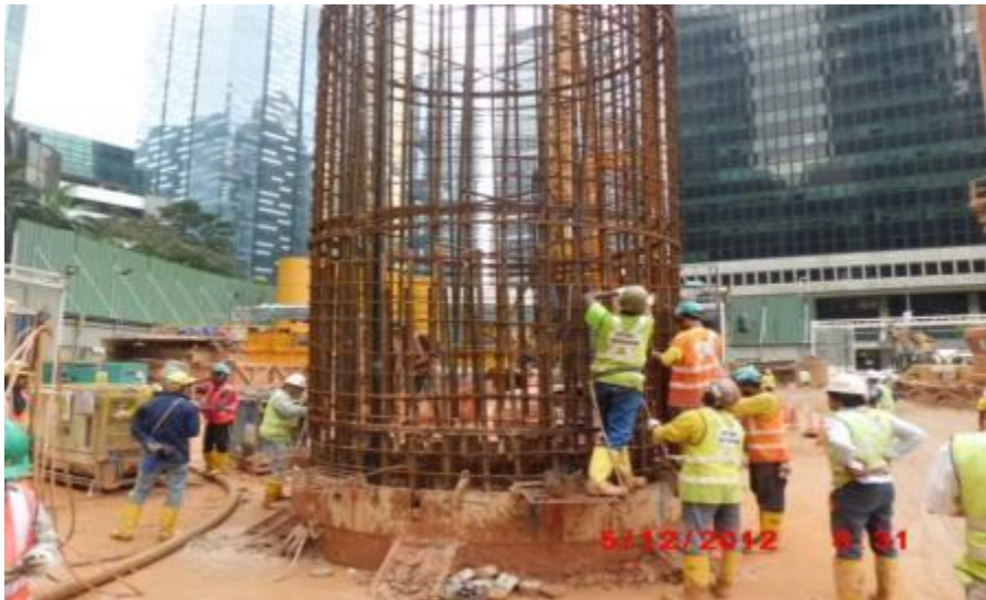
Construction of 3.5 diameter pile
