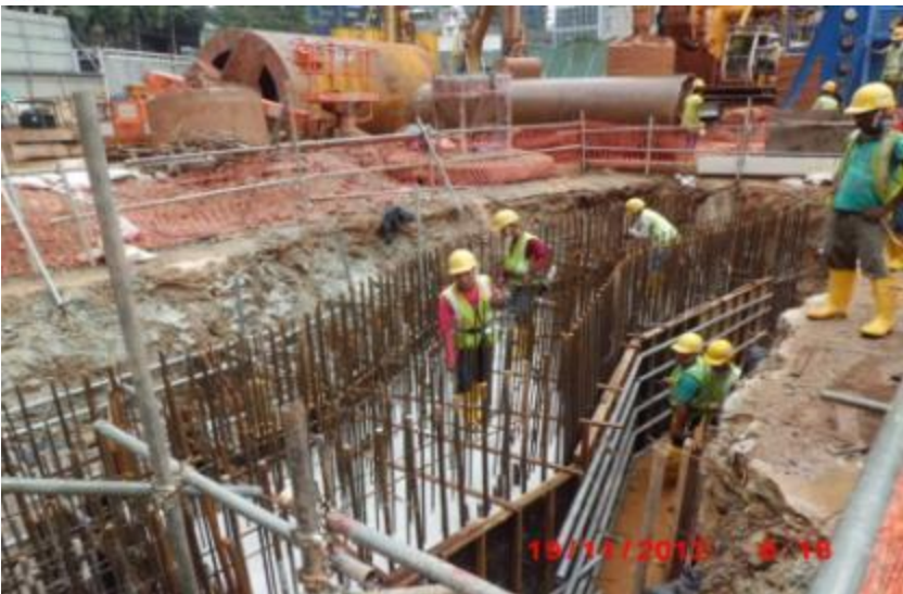
Commencement of Capping Beam
