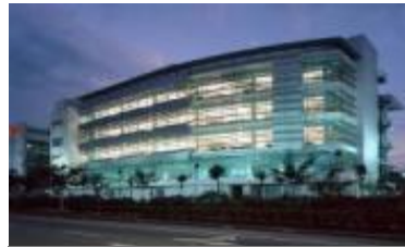
Quill Building 1 - DHL 1
