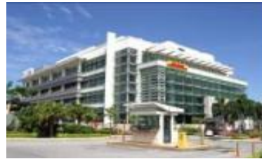
Quill Building 4 - DHL 2
