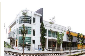
Quill Building 8 - DHL (XPJ)
